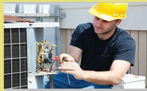
INSTALL AND REPAIR
