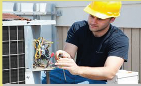
INSTALL AND REPAIR
