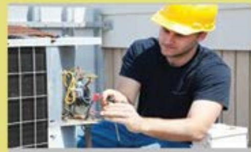
INSTALL AND REPAIR
